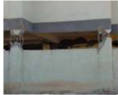
Fig 14:- Damage to buildings due to short column effect on columns
