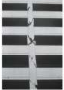
Fig 14:- Damage to buildings due to short column effect on columns
