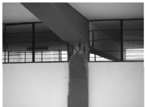
Figure 2-12 Short column failure. 2007 Pisco, Peru earthquake. (Reproduced with permission from Darin Bell)
