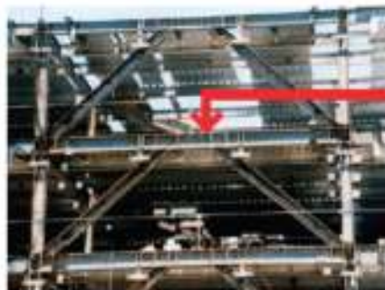
eccentric brace with link beams
